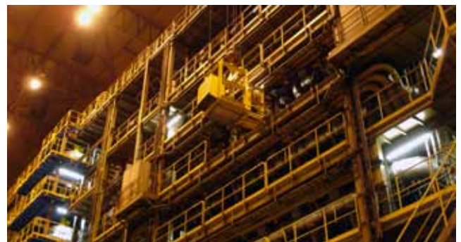
The continuous annealing line at SSAB in Borlänge, Sweden.
